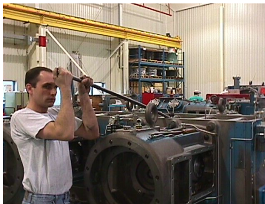
Using Pry Bar to Check Jack Clearance
