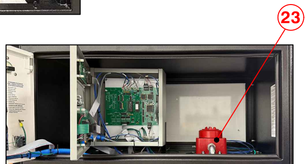
UPPER ENCLOSURE INTERIOR
